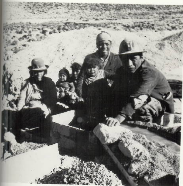
(21) Indian miners concentrate cassiterite ore, using a small stream, at Santa Isabel mine, 20 miles from San Pablo.
