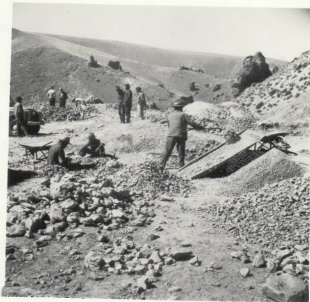
(22) Indian miners crushing and sorting ore by hand, Bolivar Mine. The vehicle on the left is the expedition's Land Rover, not the Mines
