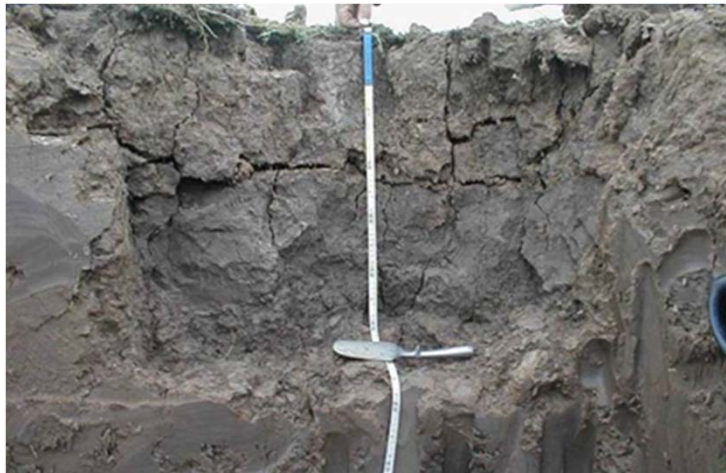
Desiccation cracking of clay embankment
