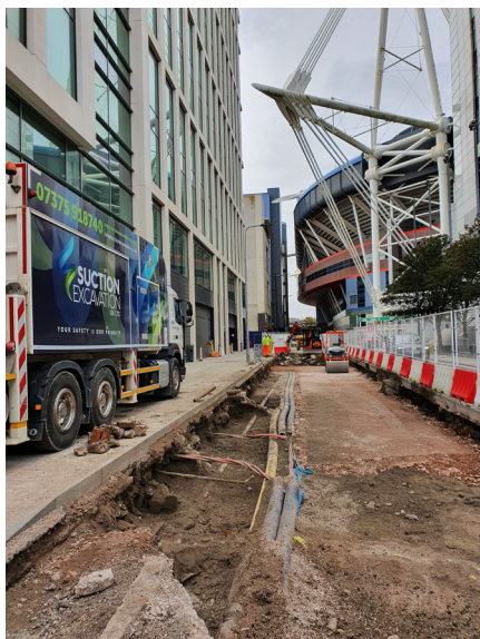
Moving utilities at the Cardiff Central Square project
