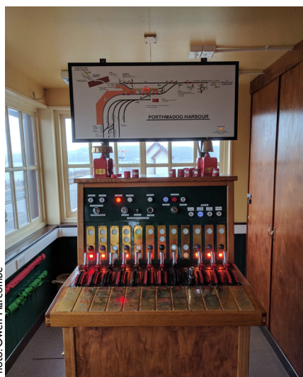
The signalling frame in Porthmadog signal box which controls signals and points in the station
