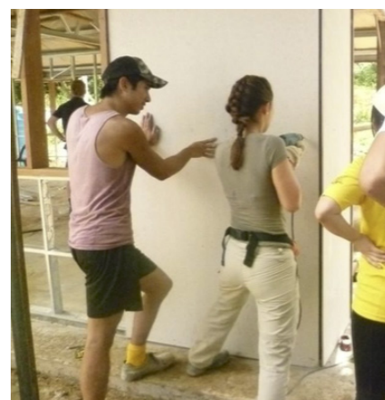
Jana drilling the cement board onto the steel frame
