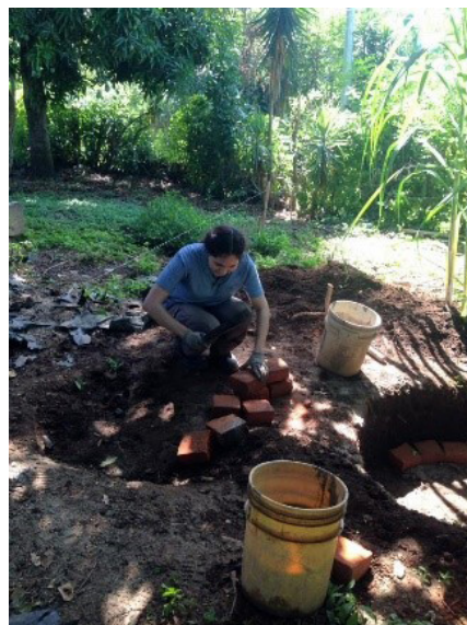
Cutting the bricks for the Pit Collar
