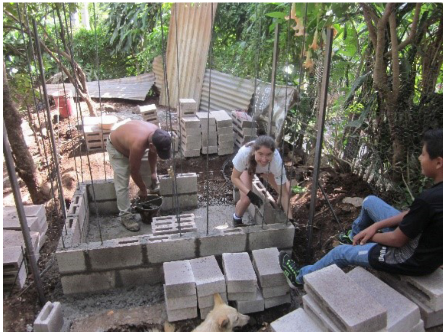
Building the two composting units
