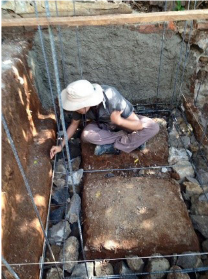
Abonera foundation trench filled with rocks and reinforcement on top
