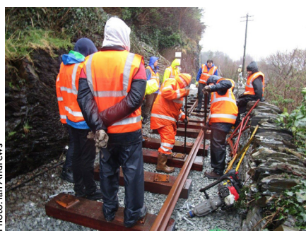
Using crowbars to ensure sleepers were in the correct place and evenly spaced
