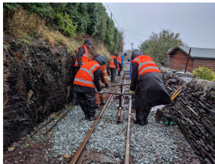
Putting the rail onto the rollers
