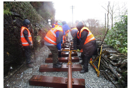
Lifting one of the new rails into place
