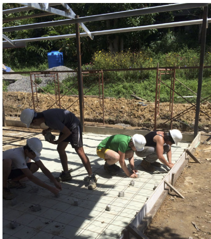
Jana drilling the cement board onto the steel frame
