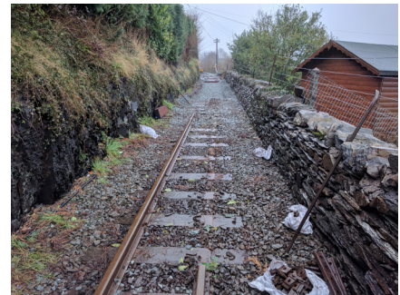
The section of track where the rail had been removed
