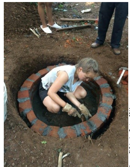
Laying the bricks
