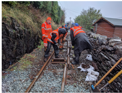
Using the rail tongs to lift off one of the old rails
