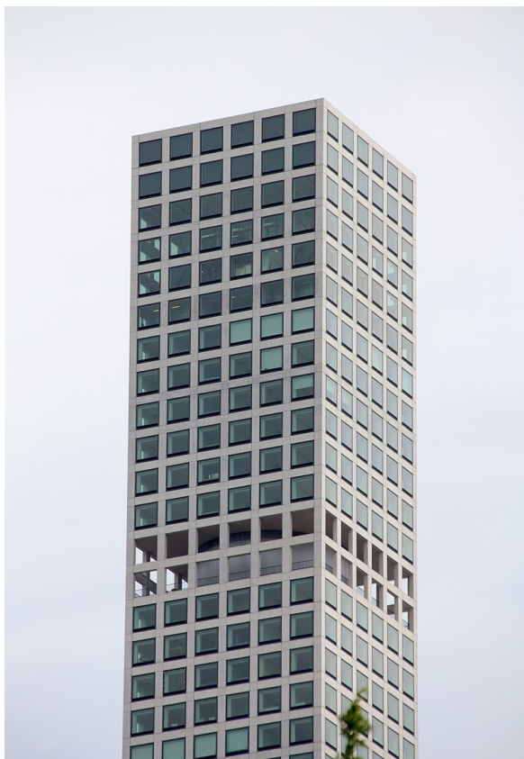
Figure 8. 432 Park Avenue, New York. This Skyscraper is divided into seven vertical segments, each with 12 occupied floors. Between each segment is a two-story open section without any windows to allow air to flow through. (Peel, 2020)
