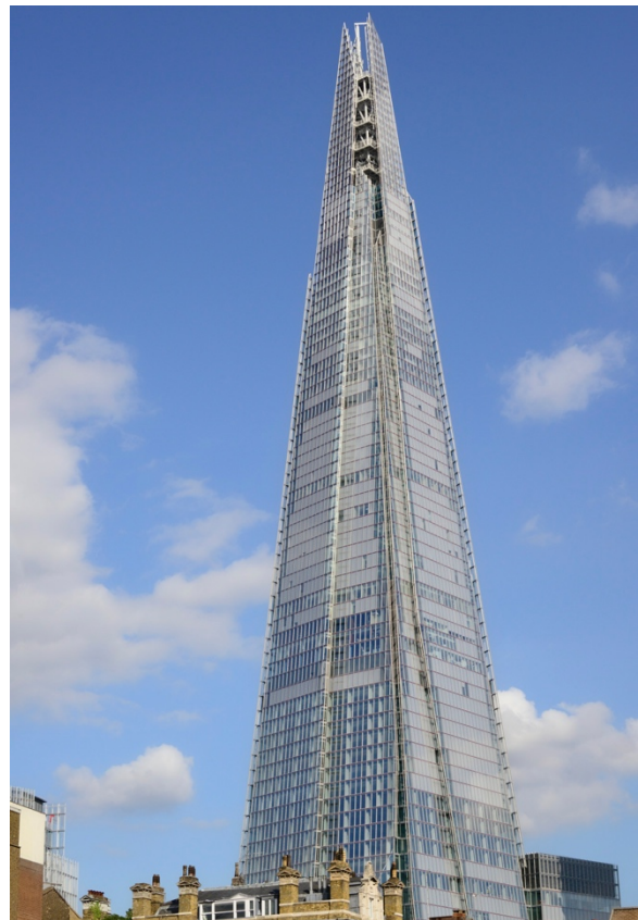
Figure 5. The Shard exploits the advantage of reducing the width of cross section along the height to minimise the wind induced vibrations at the top of the building. (ArchDaily, 2020)
