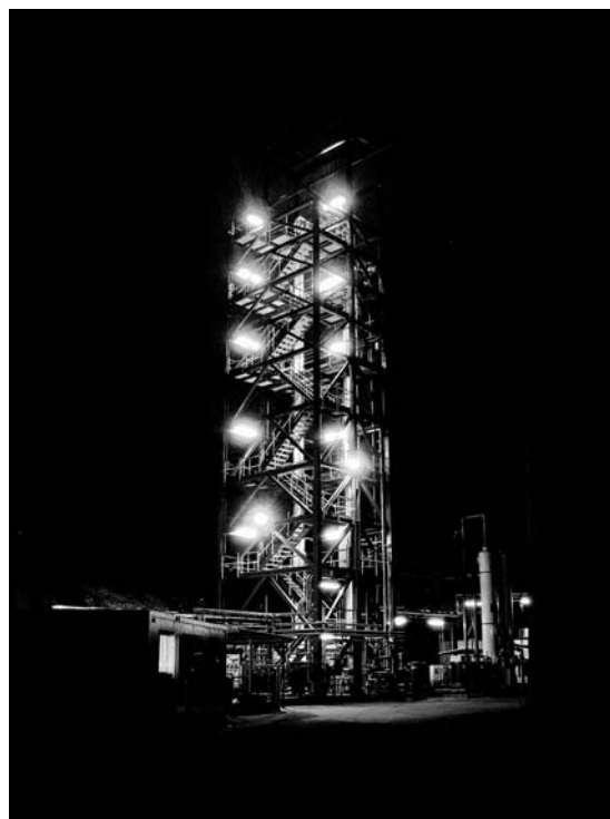
Fig. 2 Endesa’s amine-based post-combustion pilot plant. Based in the Northwest of Spain, in PC Compostilla, this plant has the capacity to treat 800 m 3 h -1 of flue gases.
