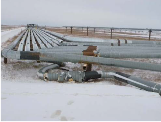
(a) The ruptured gas line
